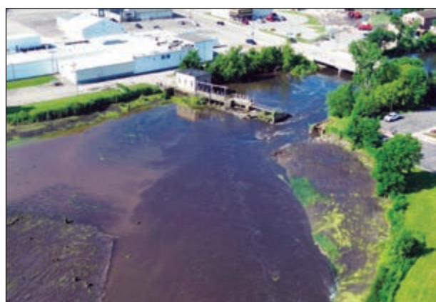
The Manawa Mill pond after the north side of the dam was breached and the Little Wolf River flooded Friday, July 5.
