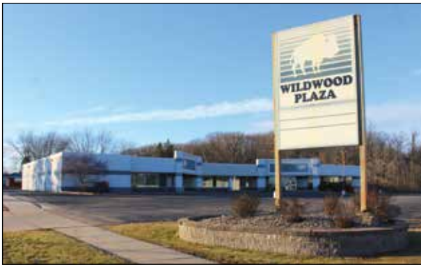
This commercial property at 2504 S. Central Ave., known as the Buffalo Building, has been identified as a possible future location for the Marshfield Police Department.
