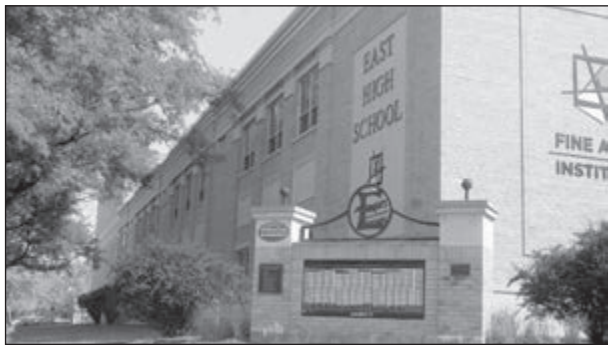
Some funding would address entrance security and bathroom renovations at East High, Edison, Franklin, Lombardi, Preble High, Red Smith, Southwest High, Washington and West schools. Kris Leonhardt photo
