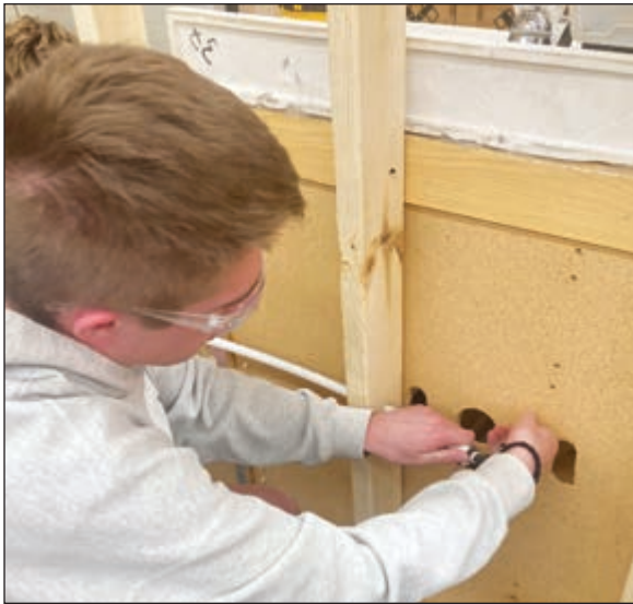
Instructor Andy Peissig thanked DM Plumbing and Sewer for the materials, tools and expertise.
