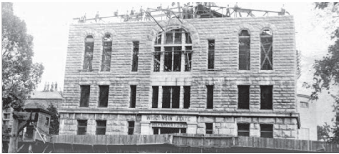
A building for 600 residents was constructed in 1898. Now 126 years later, the facility is still operational but struggles with issues of overcrowding and understaffing. Green Bay Correctional Institution photo
