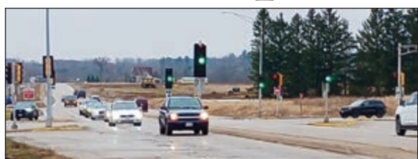
Intersection of State Highway 15 and U.S. Highway 45 facing south in Hortonville. John Faucher Photo
