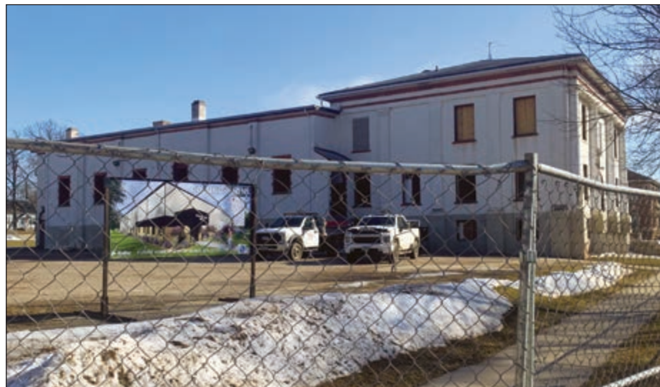
The former Armory will soon be the site of a new Clintonville Utilities building. Jeff Hoffman Photo
