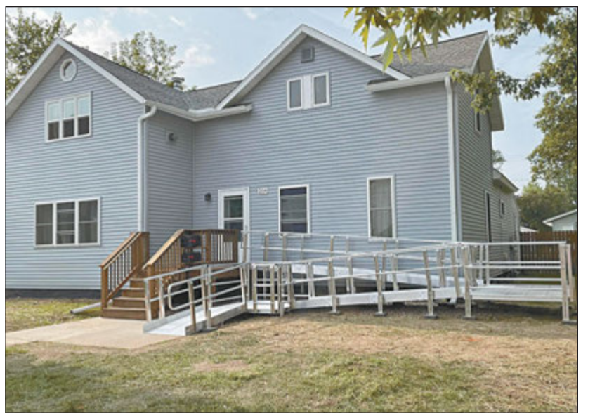
After: All new windows, new siding, new soffit and fascia, a new front door and porch, and a handicap accessible ramp make their home maintenance free for many years to come and more easily accessible for Jacki.
