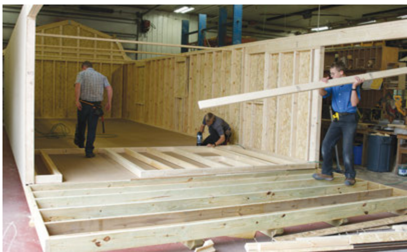
Employees at Baker Barns constructing a new building in the shop.
