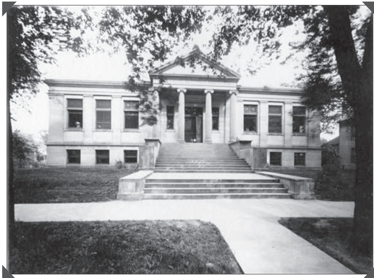
An exterior view of the Green Bay Public Library. The “Carnegie Library” was built in 1903 with donated funds from Andrew Carnegie. Around 2,500 of these libraries were built 1883-1929 — most in the United States and UK.
