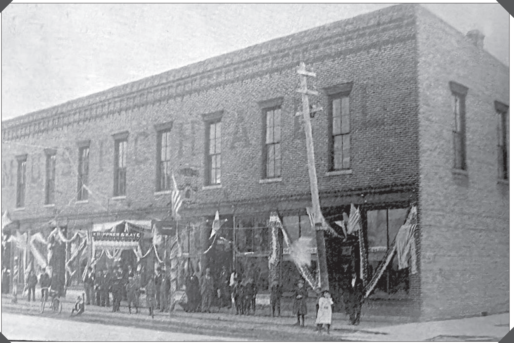
Letters arranged in the brick spell out MUSIC HALL on the front of this building which was located at 409 West Walnut St., Green Bay, on the corner of Walnut and Maple Avenue. It was built in 1882 in a commercial vernacular architecture style and served as an opera house and concert/dance hall on the second floor, while the first floor was leased to businesses. It was demolished in 2010. Neville Public Museum of Brown County photo
