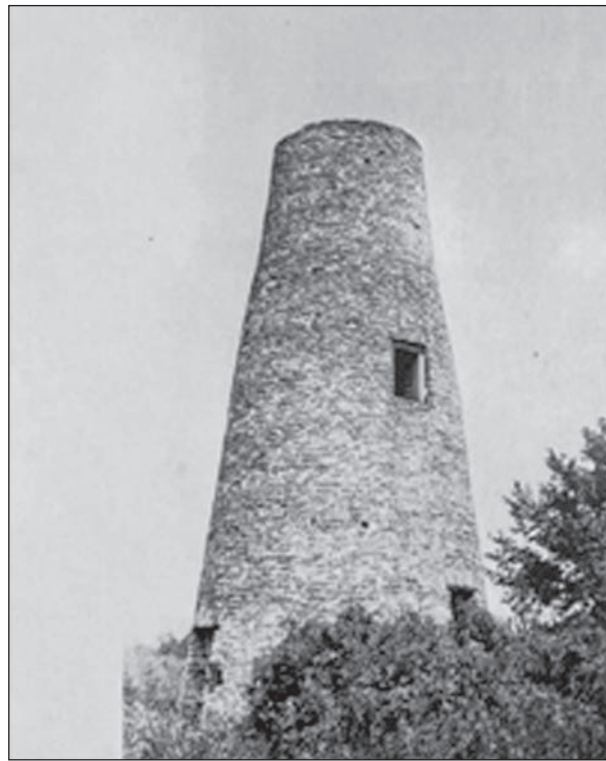
Long Tail Point's first lighthouse built in 1847. It was built using sand and limestone found on the eastern shore of Green Bay.
