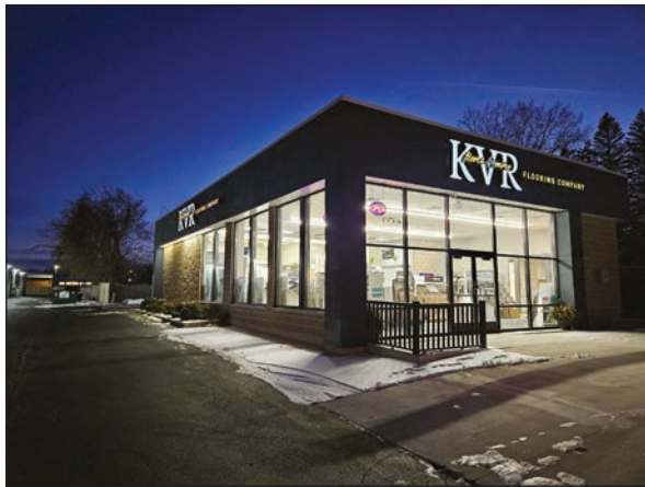
This store, which expands upon the flooring business Van Rixel already had, focuses on providing an array of flooring products in addition to installation services. Submitted photo
