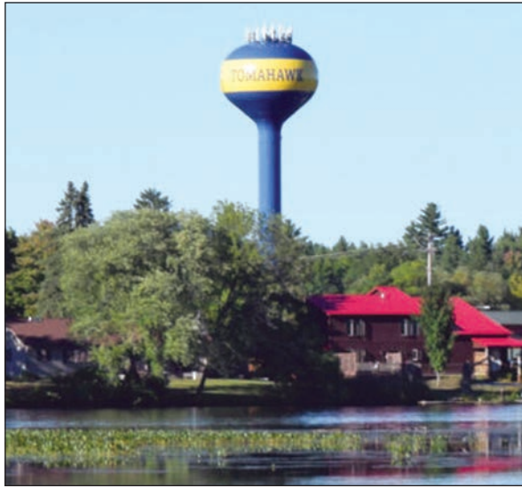
The City of Tomahawk's water tower is in the running for Tnemec Company Inc.'s Tank of the Year award.
