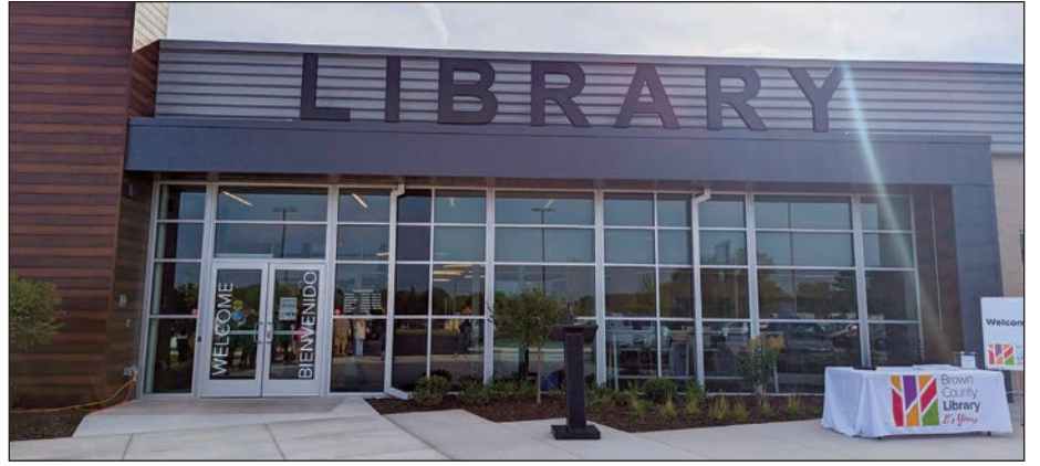
The new East Branch location of the Brown County Library is directly next door to the old East Branch, at 2253 Main St. in Green Bay,
