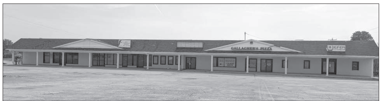
Allouez will move forward with razing the building at 1905 S Webster Ave., formerly home to Gallagher's Pizza, to make room for future development. Janelle Fisher photo
