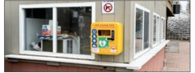
The AED device is now mounted in a secure cabinet on the outside of the concession stand at Merrill's Athletic Park, where someone can call 9-1-1 to report an emergency and then get immediate access to the defibrillator to perform life-saving measures until paramedics arrive.
