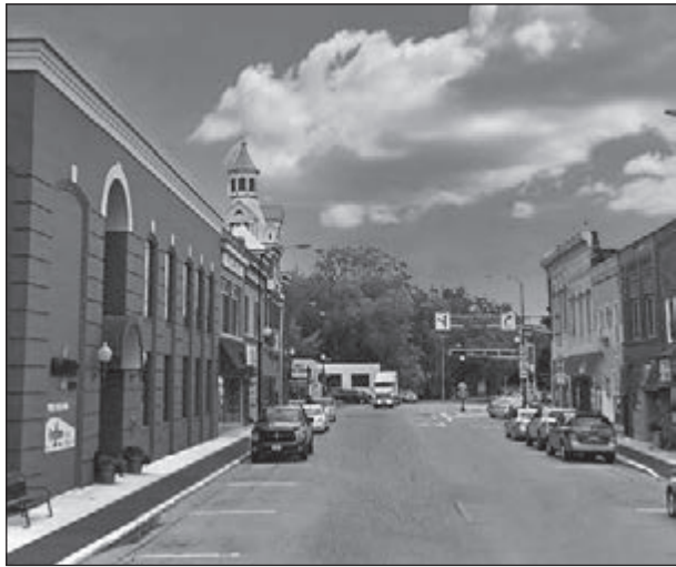
North Water and Pearl streets a continuous dark gray with a brick pattern in select areas.
