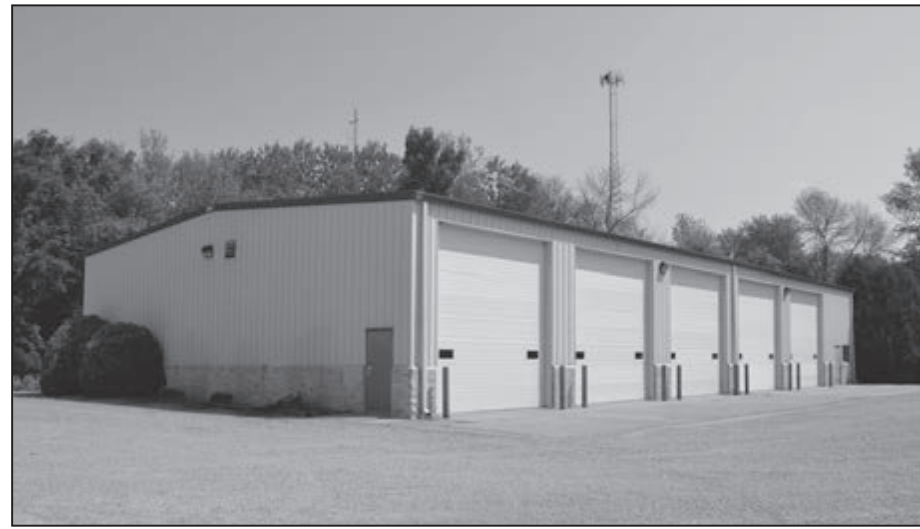
The Fremont-Wolf River Fire Department has a new building on 600 W. State Road 110 near Ma's bait & Tackle. Chief Miller said transforming the building into an operational fire station is a work-in-progress and there is much work to be done.
