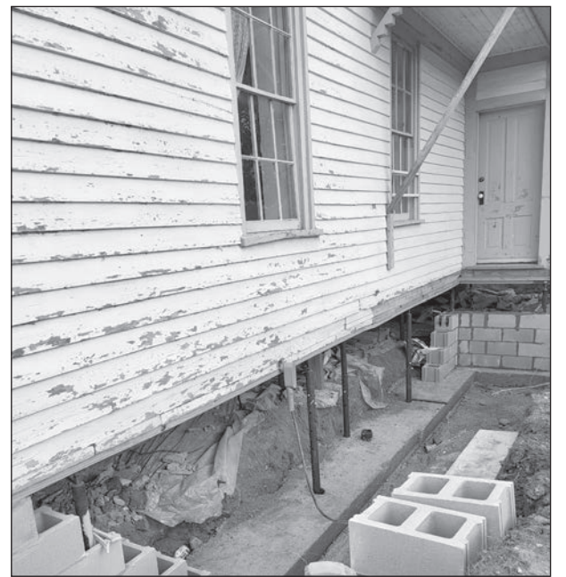
Before-and-after photos of the historic Cordwood House in Clintonville during reconstruction of its foundation.
