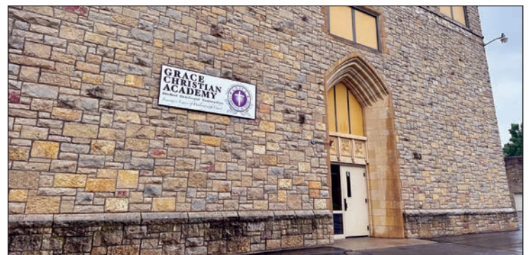
GCA’s new property in Green Bay is located at the Annunciation school facility, where Providence Academy was previously located. Kris Leonhardt photo
