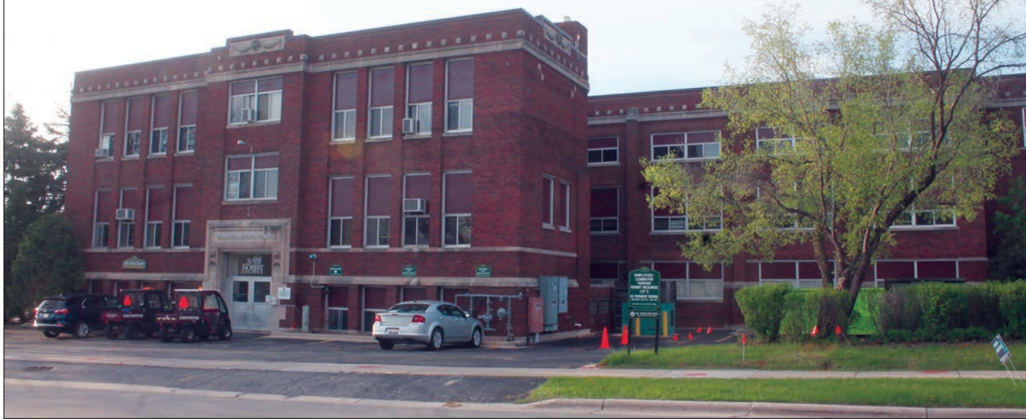
Pennings High School was constructed as Nicolet High School in 1923 and became part of the West De Pere School District. Kris Leonhardt photo
