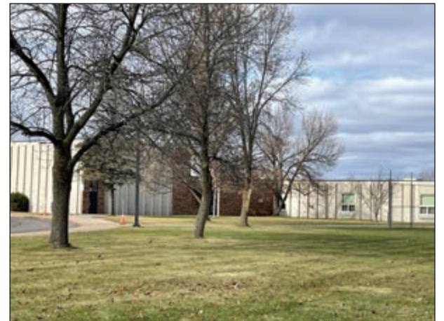
The Jefferson Elementary School building and grounds. Tina L. Scott photo.
