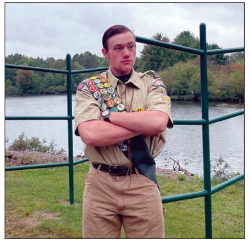
Stefanich's Eagle Scout project was the construction and installation of a canoe and kayak rack at Bradley Park. Photos courtesy of Susan Stefanich
