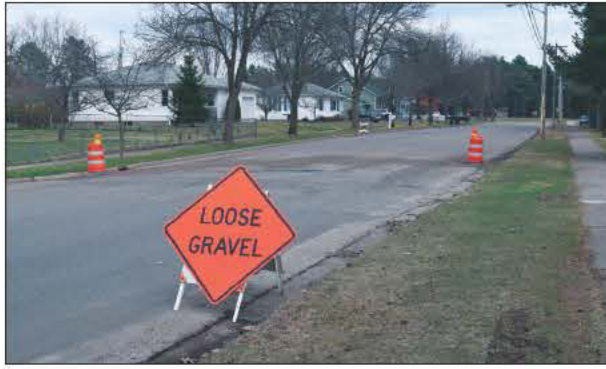
The location of the deteriorating culvert on Lincoln Ave., behind Pride Park. Photo by Jalen Maki
