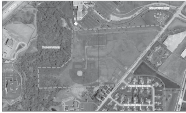
Kingston Preserve development is in the 2000 block of Lawrence Drive, southwest from the intersection with Employers Boulevard. City of De Pere image
