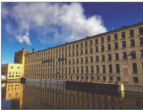
The Nicolet Paper Mill, currently owned by Ahlstrom-Munksjo, has been a De Pere landmark since 1892. Rick Cohler photo
