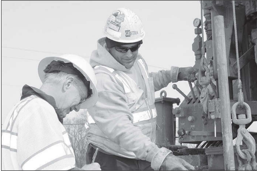
WisDOT workers look at type of soil, bedrock depth and groundwater conditions for state roadway infrastructure. WisDOT photo
