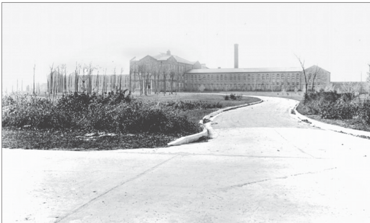
In the final months of 1901, foundation for the addition was going in as reformatory staff was dealing with a new challenge.
