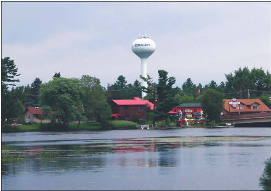
Tomahawk's water tower is slated to get a facelift later this year. Photo by Jalen Maki
