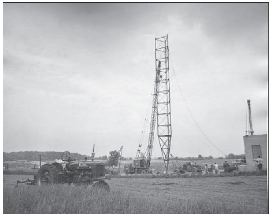
The transmission tower under construction north of Oconto.
