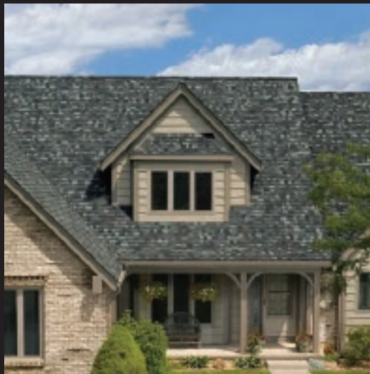
STORM DAMAGE EXPERTS
