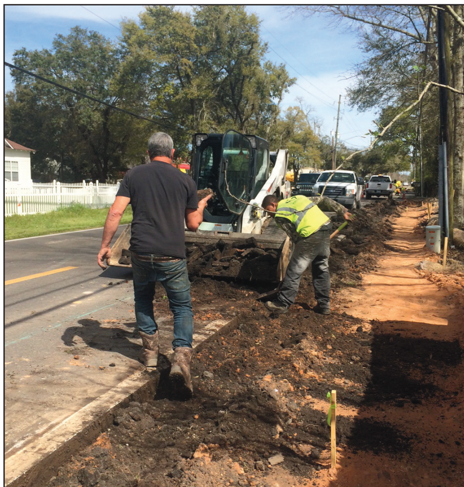
Preparation for sidewalk
