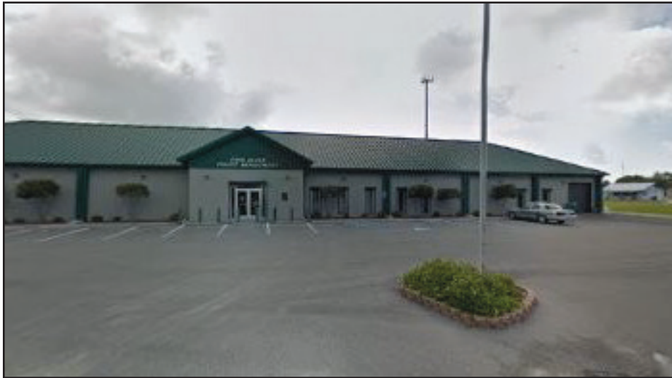
Long Beach Police Headquarters 201 Alexander Road
