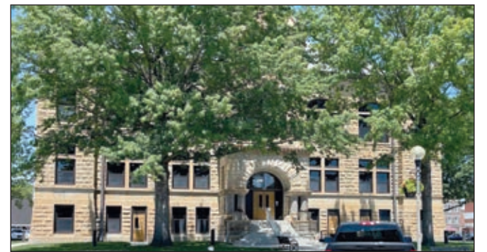
Adair County Courthouse
