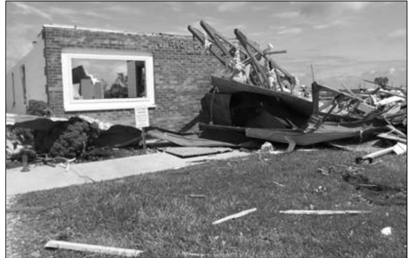
The post office in Baring was destroyed by an E2 tornado.
