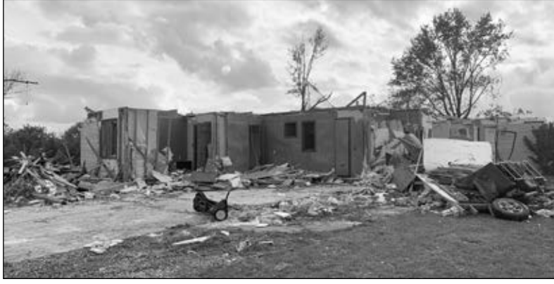
A home in Baring that was damaged by an E2 tornado that touched down on the late evening of Aug. 4.
