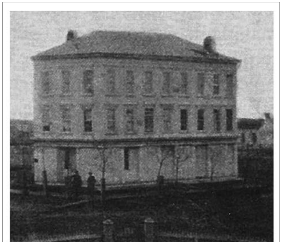
Linder Building on the southeast corner of the Kirksville square, built 1858 by William Parcels Linder (1819-1884)
