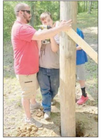
Tyler Lynak assists Cormac Nolan in setting the poles plumb while Nolan secures the temporary bracing.
