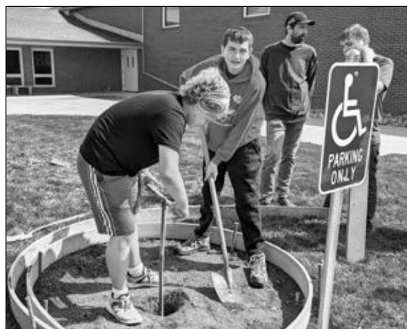
Second Class Scout Drew Mayes and Life Scout Conner King dig the base for a flag pole and clean up inside the formwork.
