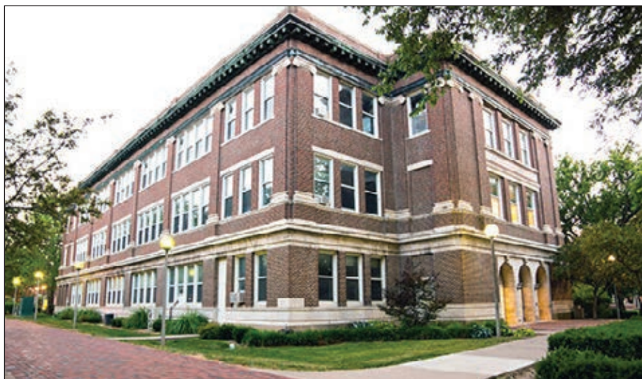
Truman State University will renovate the Kirk Building to house a new Student Success Center to be utilized by Truman students as well as a Sustained Knowledge of Integrated Lifelong Learning Skills (SKILLS) Center for area K-12 students, non-student community members and other adult learners.
