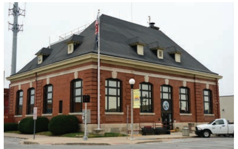
Kirksville City Hall, which is a historic landmark in the city.
