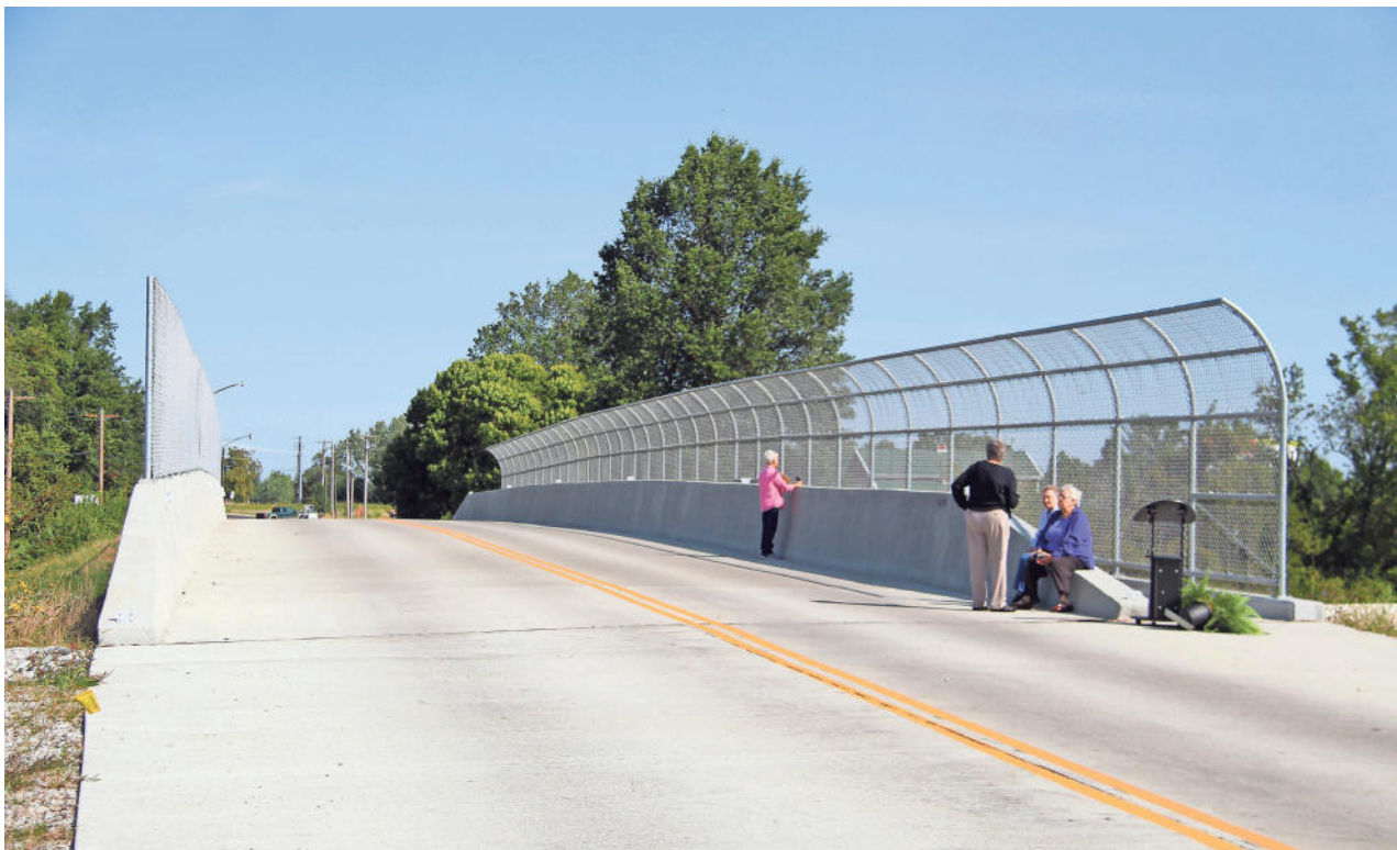
The Lester Dent Memorial Bridge in La Plata. AUSTIN MILLER
