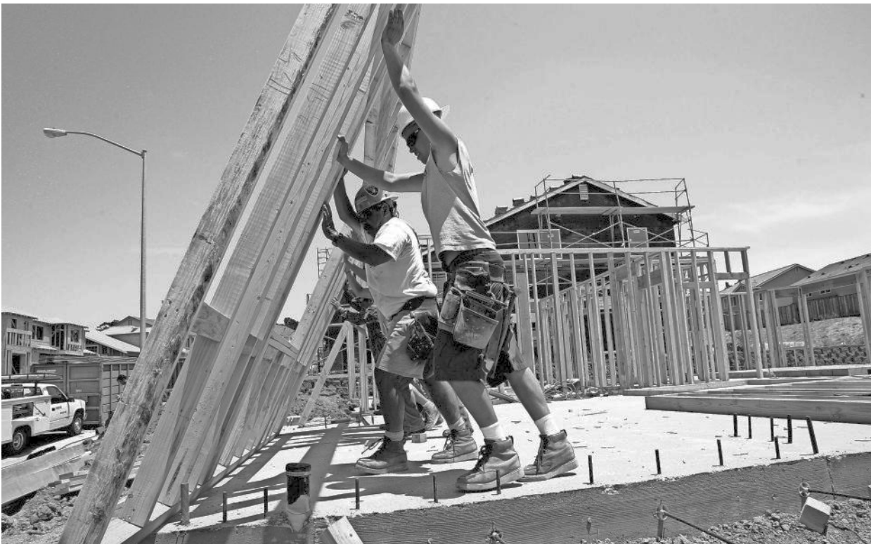
Construction workers raise wood framing in a new housing development. JUSTIN SULLIVAN/GETTY IMAGES
