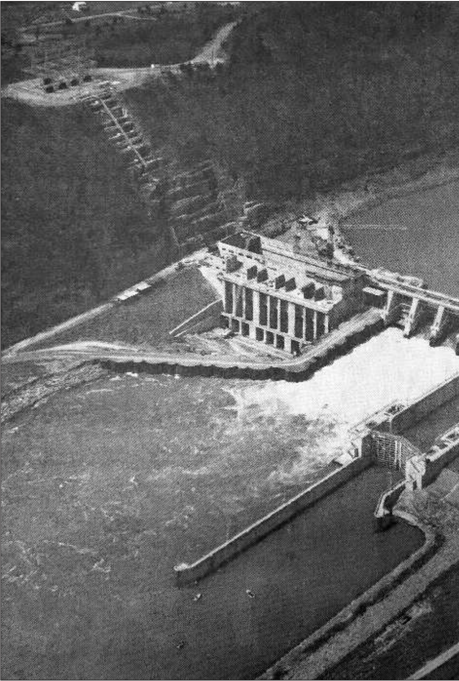
Lock And Dam – The aerial view of Cordell Hull Lock and Dam, located on the Cumberland River near Carthage, shows the status of construction of the powerhouse. The lock and dam is complete and the impoundment for the reservoir is scheduled for this fall. The power plant will have three units with a total of 100,000 kilowatts generating power. The powerhouse construction is 69 % complete and is scheduled for overall completion in December 1973, but the first generating unit is scheduled to go “on-the-line” early next year. (From the April 27, 1972 edition of the Jackson County Sentinel)
