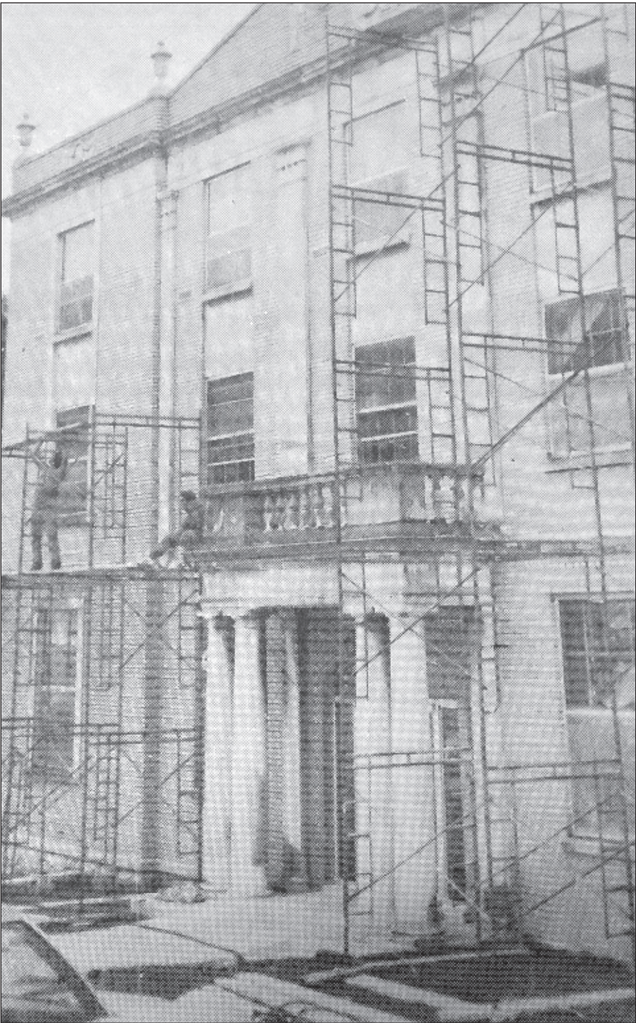
Repairs Set – Scaffolds were erected last Thursday and Friday for repair work to begin immediately on the concrete outside the Jackson County Courthouse. The crumbling of the concrete on the structure is partially caused by the hard freeze during the past winter, officials said. (From the June 20, 1985 edition of the Jackson County Sentinel )
