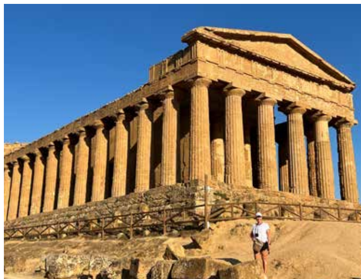
The Valley of the Temples in Agrigento, Sicily, is a stunning example of ancient Greek architecture.
