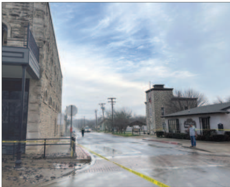
Debris from the fire was "everywhere," according to Paula McDonald, who owns two businesses near the Nutt House Hotel.
