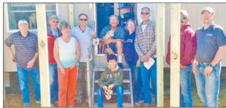
GIVING SPIRITS: Members of the Hood County Builders Association pose for a photo after participating in a recent Hard Hat Helpers project in which they built a porch and a wheelchair ramp for a disabled man.
