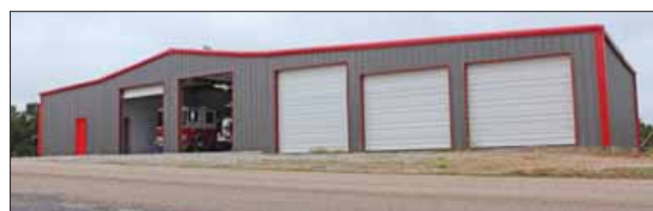
FINAL PREP: Last minute painting is underway at the renovated and expanded Station 70 in Oak Trail Shores before the open house on Oct. 7.
