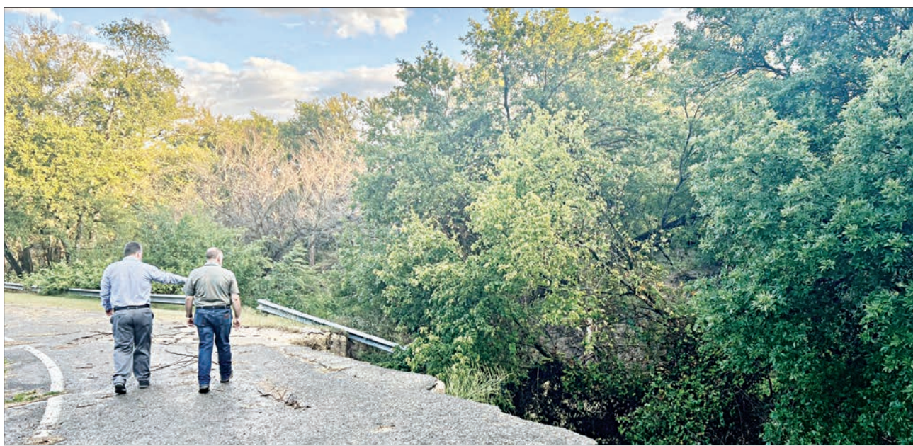
Top photo: Trees and other debris litter the Leon River around Faunt Le Roy Park, left behind from flooding in May and June. Bottom photo: City of Gatesville Financial Supervisor Mike Halsema (left) and Councilman Greg Casey assess the damage to the roadway around the park as a result of the river bank deteriorating.
