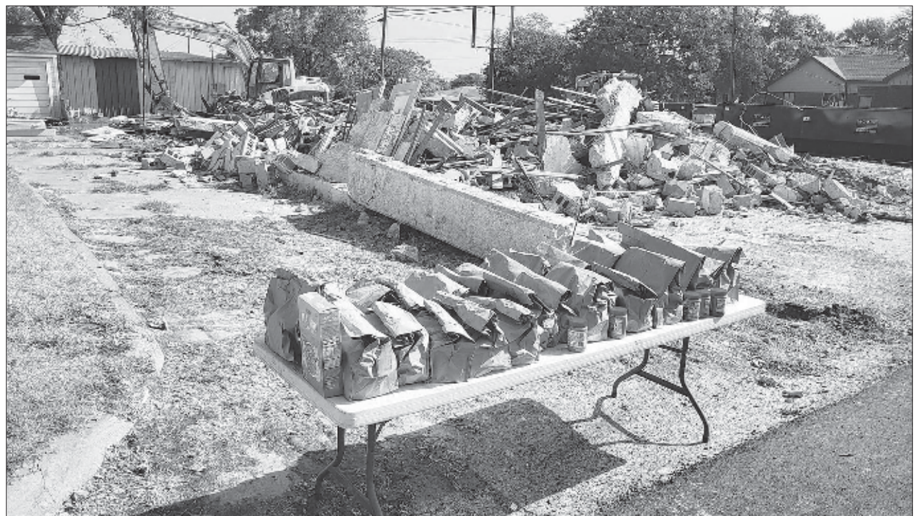
Demolition site of where Mission Gatesville's building once stood on Lutterloh.
