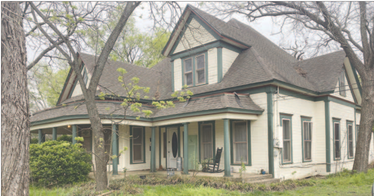
A home on College Avenue in Oglesby can be traced back to a catalog "home-kit" that was ordered and assembled on the spot.
