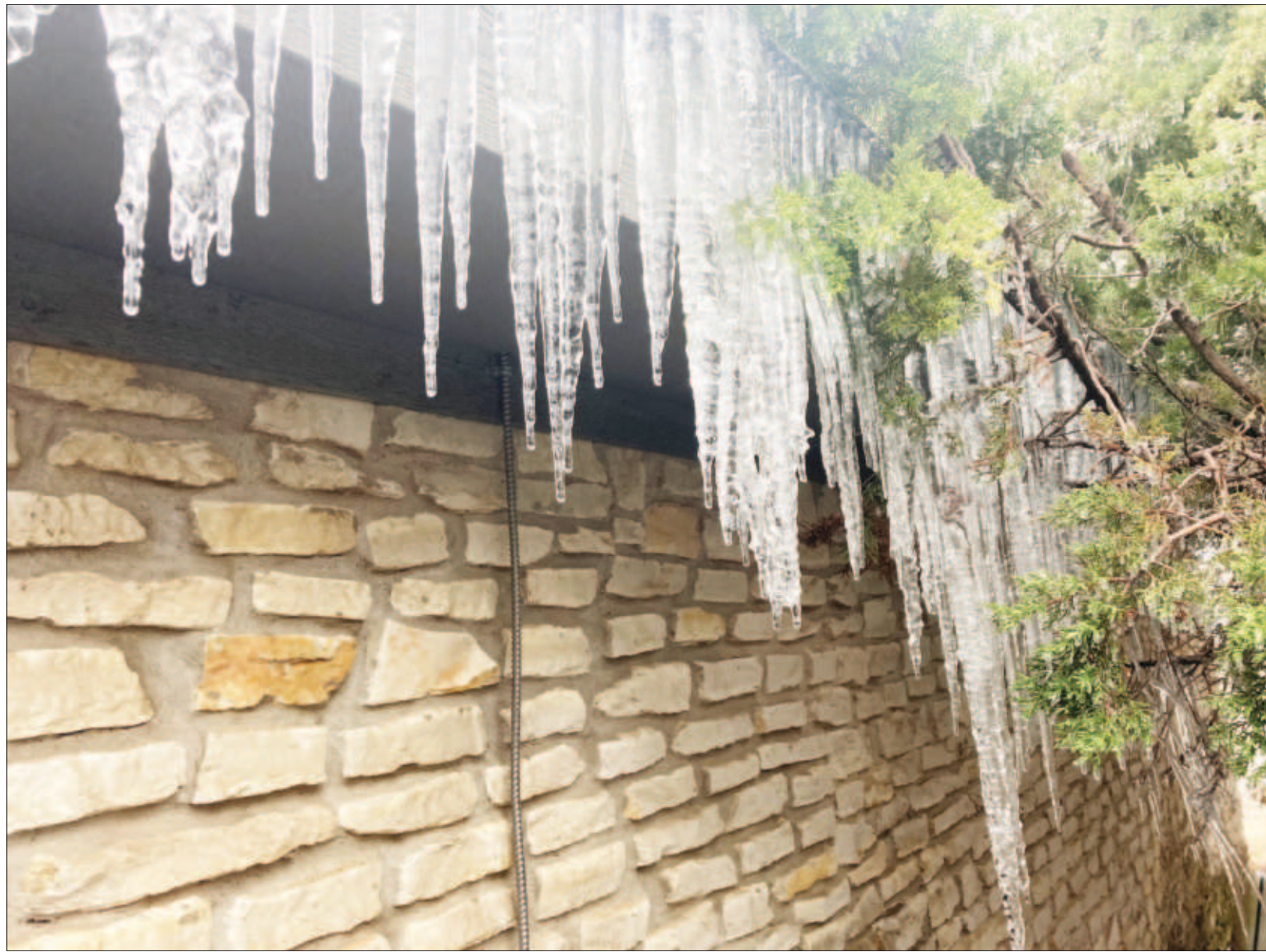
Icicles of varying lengths hang off a house east of Gatesville in the Pecan Grove area. Freezing weather had a big impact on the area, resulting in the closure of local schools for three consecutive days, Jan. 31 through Feb. 2.
