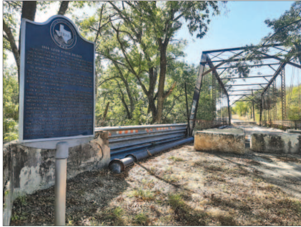
1904 Leon River Bridge
