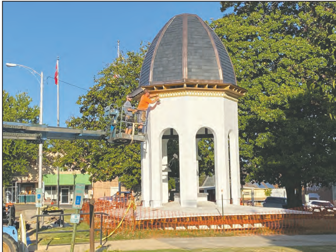
Construction work continued on the courthouse bell tower on Monday.
