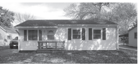
713 E. 12th Street South Sioux City, NE $179,950
